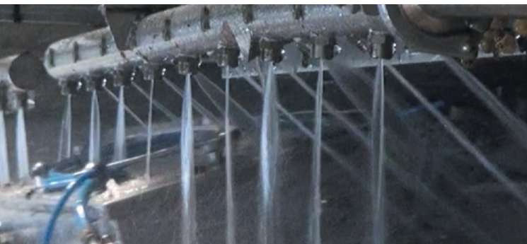
Doors spray manifold
